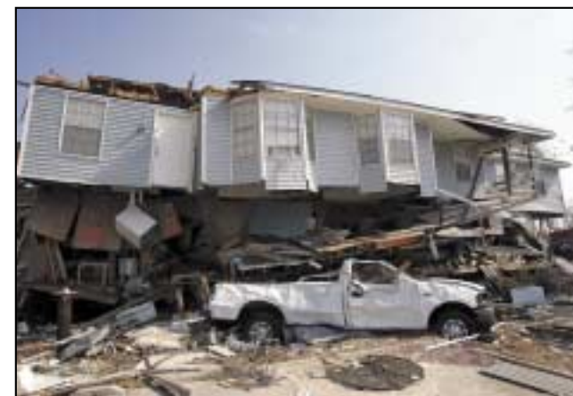
A home destroyed by Hurricane Katrina, September 9, 2005.
